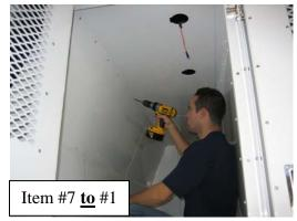
With unit positioned according to measurements on previous page, predrill and attach a #10 x 1" sheet metal screw to hold the rear **Bulkhead** in place while assembling the remainder of the unit.
